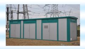
**FACTicer** uses the three phase power provided in substation to break ice on the transmission line. The power can be 35kV/69kV, 50/60Hz, 40 MW.
